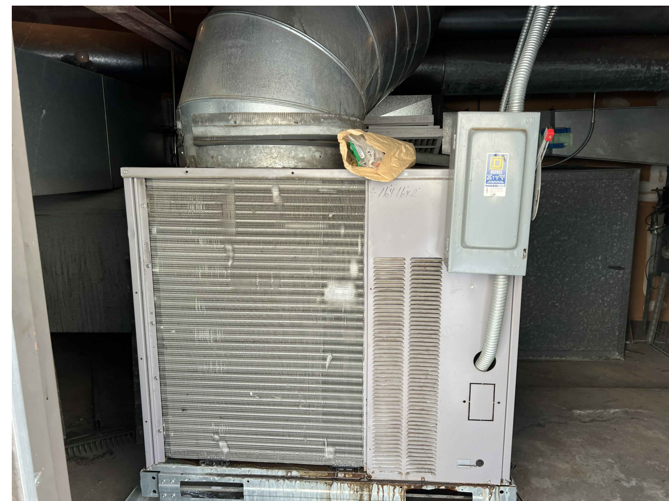
1 TYPICAL ELECTRICAL DISCONNECT @ HEAT PUMP
