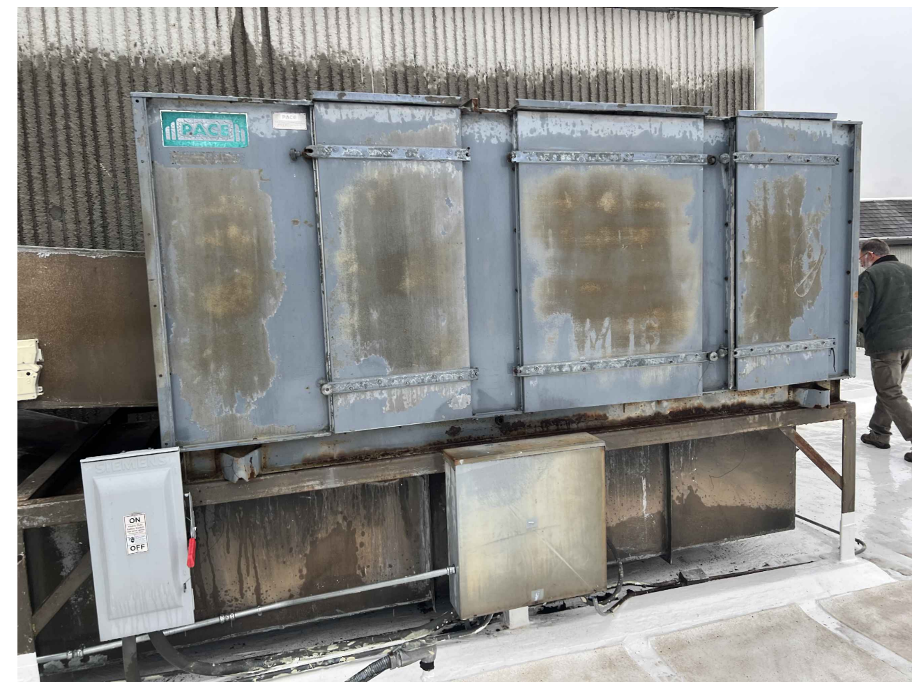
2 MD1.3 EXISTING GYM (SOUTH) AIR HANDLING UNIT (AHU-1B)
